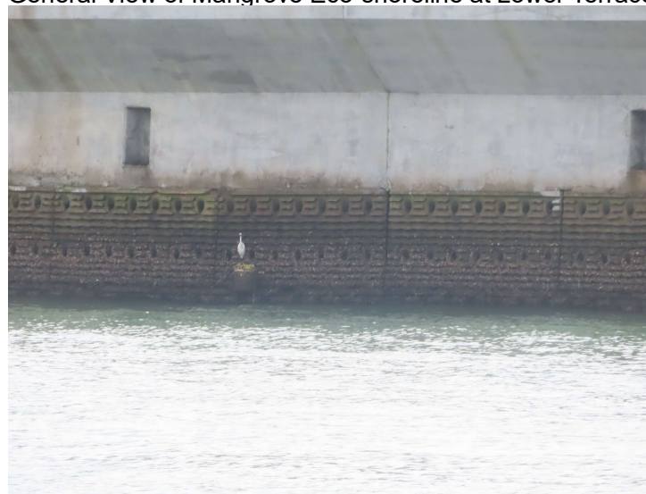
General View of Vertical Eco-shoreline
